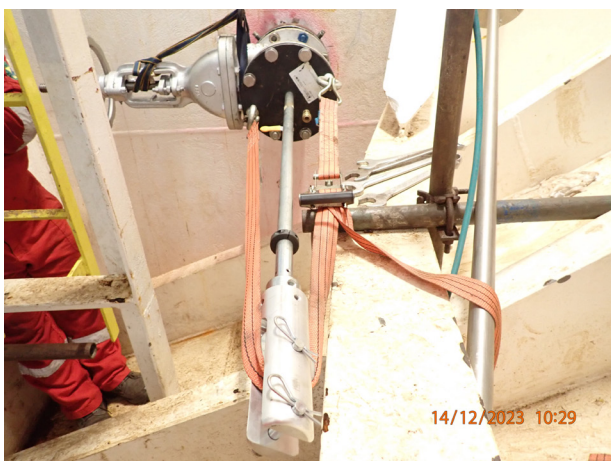
Figure 3. ODIN camera insertion for sea chest inspection during normal operations.
