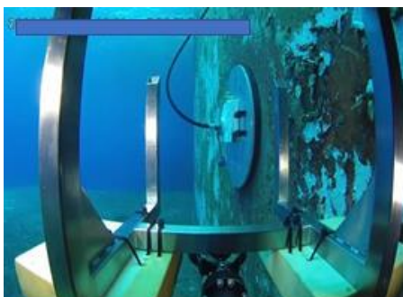
Valve Isolation with ROV Deployed ODIN Plug
