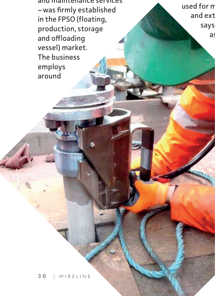
Lokring flanges installed on site
