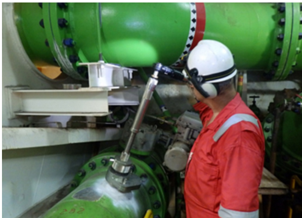
Figure 5. Camera insertion through ODIN access port.
