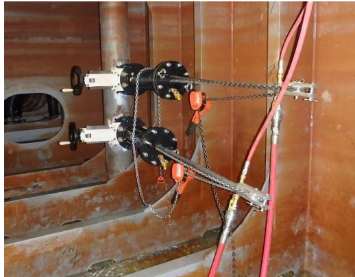
Bladder repair using ODIN inspection tool
