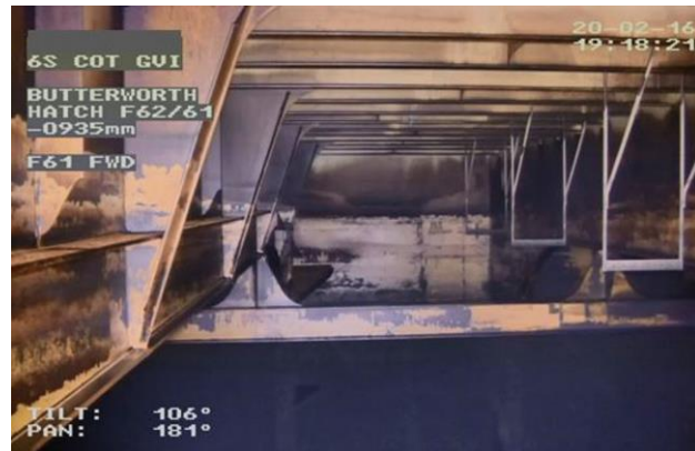
Remote optical inspection of cargo oil tank
